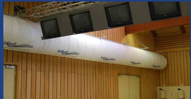
Actual diffuser with rings and no air supply
